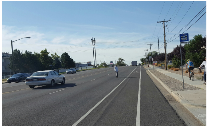
1900 West roadway conditions given a "poor" safety rating by UDOT. Conditions include unprotected bike lanes, limited street tree cover, and long distances between pedestrian crossings.
