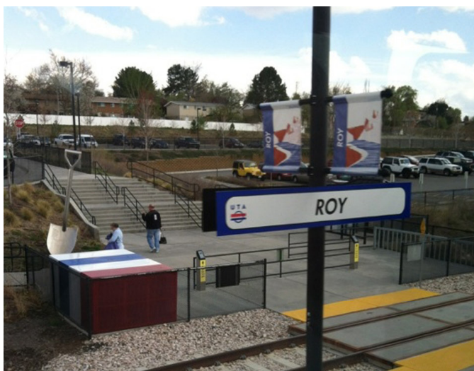
Roy FrontRunner Station
